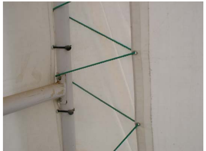
Rope Lacing Main Cover Front-Back
