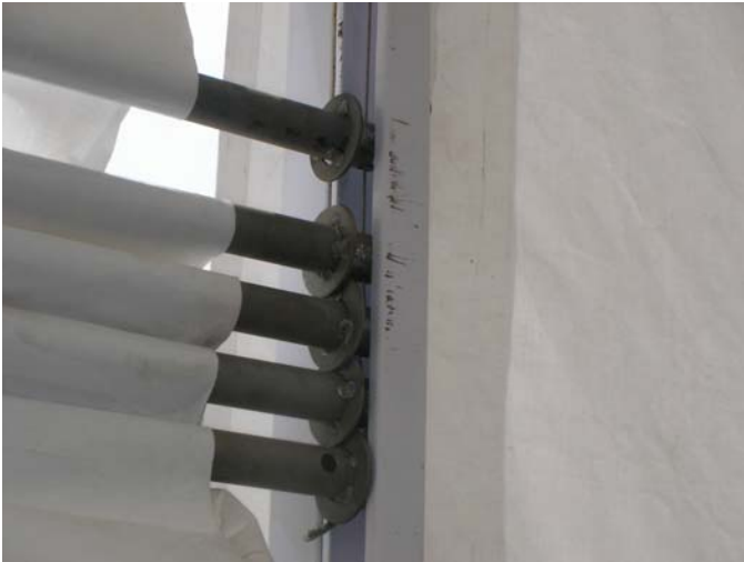
Door Tubes Inserted Into Door Track
